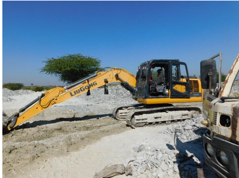
(Excavator, screen guard to be fitted from all the sides)
