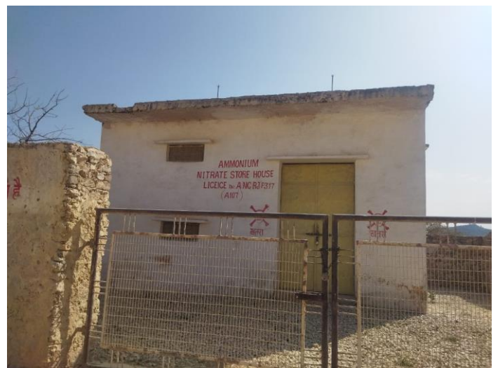
(Ammonium nitrate store house at site)
