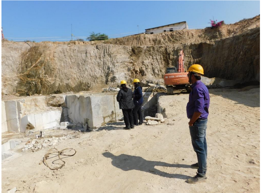
(i-Catalyst Trainer- watching the activities at site)
